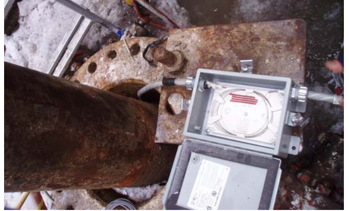
Mallik 2L-38 DTS splice in progress
