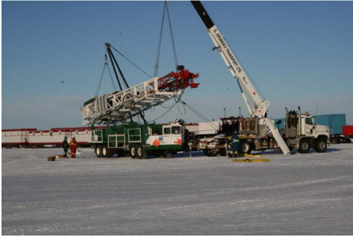
Derrick being lifted onto carrier unit
