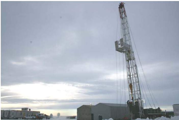
Derrick being raised
