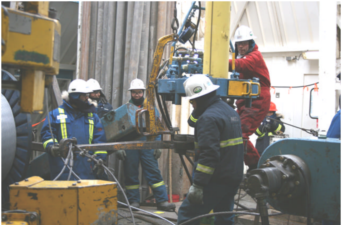
Photo of the week: Mallik 2L-38 yellow jacket casing run with 5 monitoring cables
