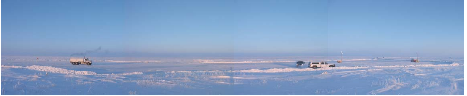
Photo montage of Mallik lease area looking northwest. Camp area is to left, main operations area including Mallik 2L and 3L well site is to the right, 30,000 m 2 of pad area will be required with an average of 20 cm of ice cover. Status as of February 11 th could not be better: Camp area 100% complete; 3L Pad area 100% complete; 2L Pad area 90% complete; Flare Pad 3 days to go.
