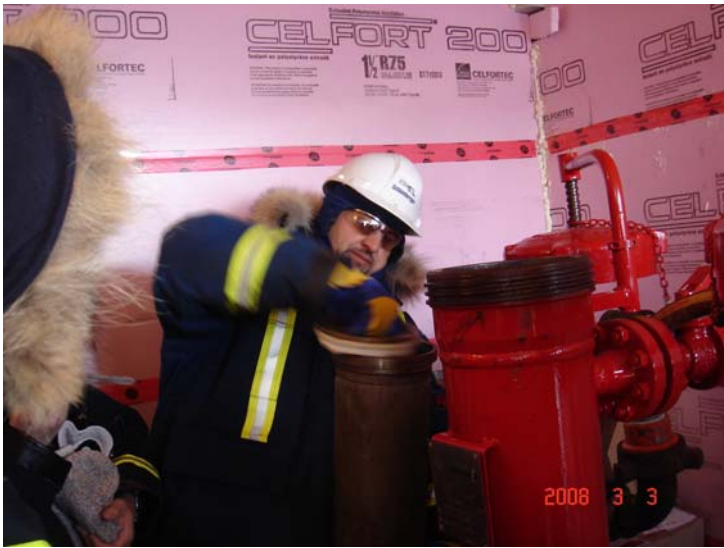
Kamel opens sediment filters from A-train
